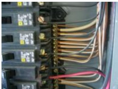
note neutral and ground wires (different sizes) under one screw
