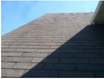
left front roof
