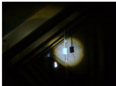
power vent thermostat and switch box....not connected
