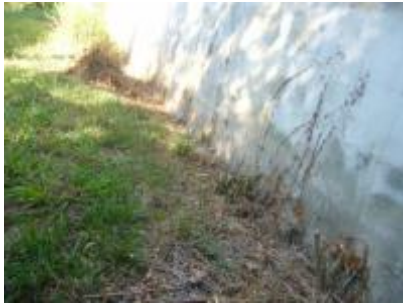
right foundation wall
